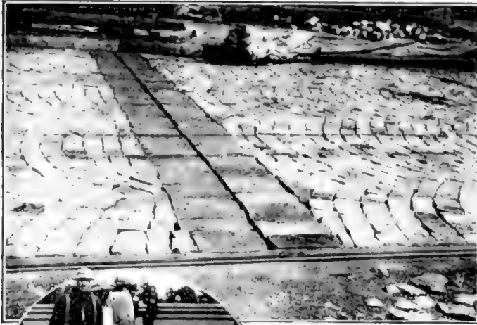
The new type of granite block pavement is laid in concentric interlocking rows, called the oyster-shell pattern
